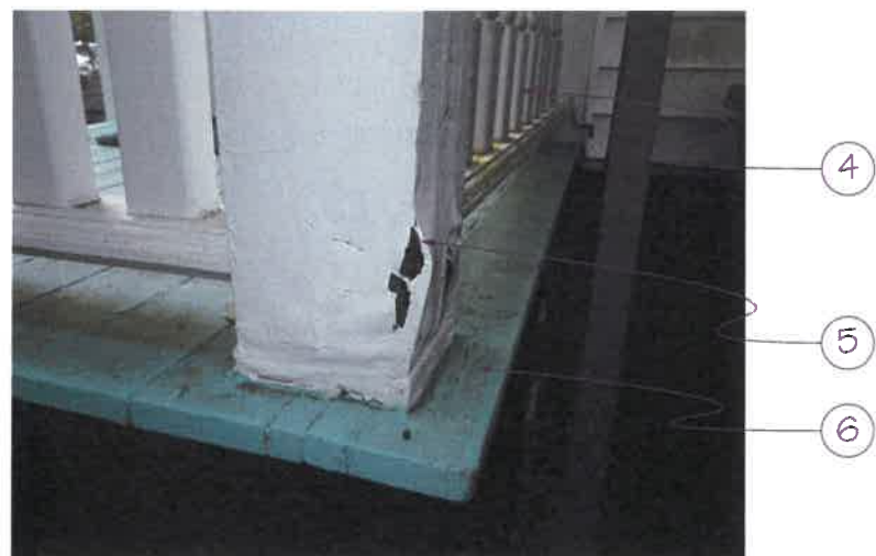
EXISTING REAR PORCH
