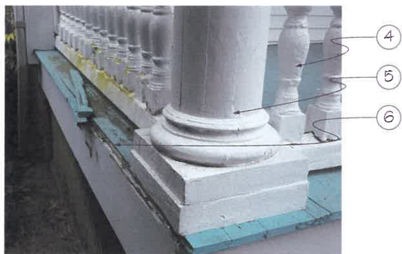
EXISTING FRONT PORCH
