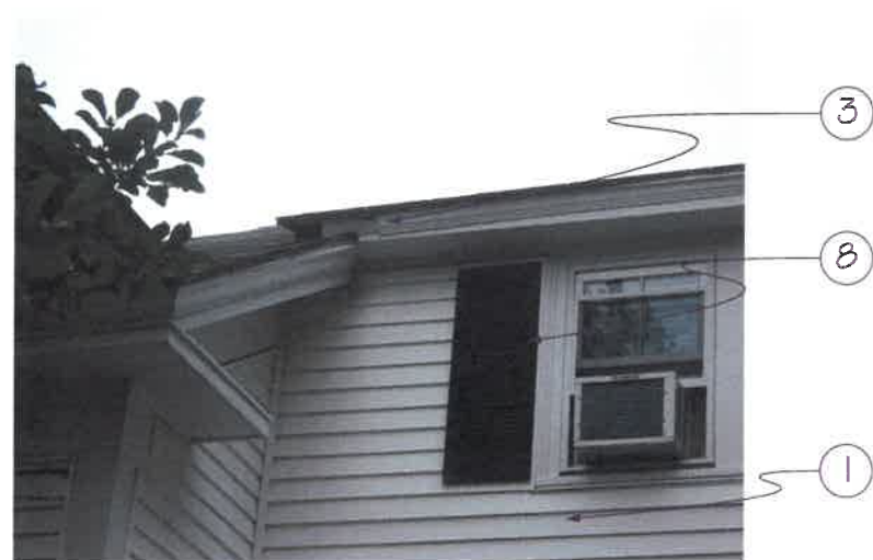
EXISTING EAVE SOUTH (RIGHT) FACADE
