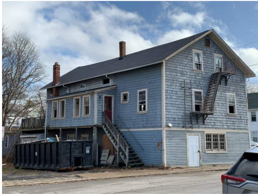
Photo #2 – North & West elevation - View from Duke street
