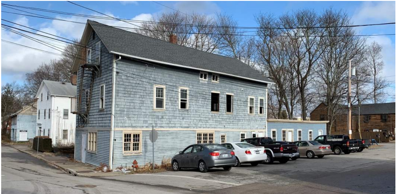
Photo #1 – South & West elevation View from the intersection of Duke Street & Queen Street
