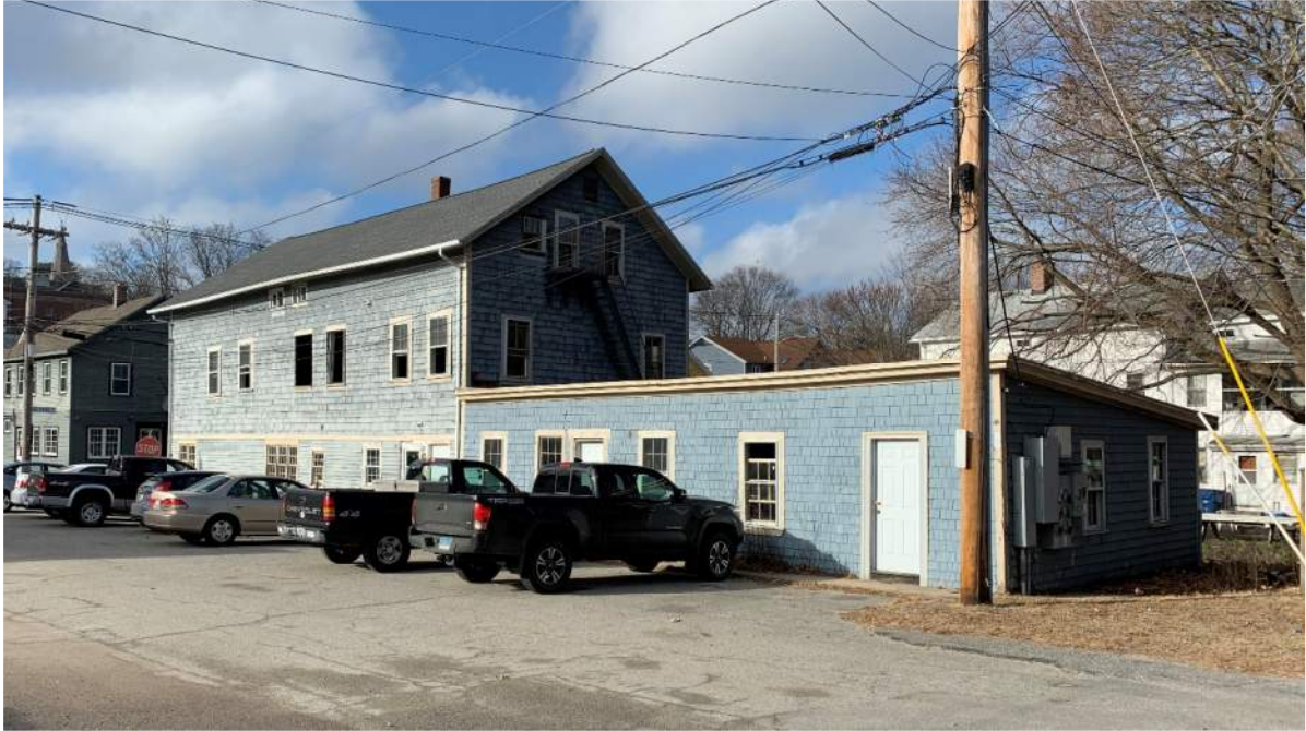
Photo #4 – South & East elevation - View from Queen Street
