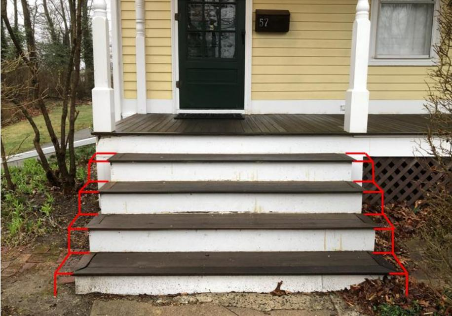
Red lines indicate new front steps (~7.5" on both sides) to accommodate porch railings
