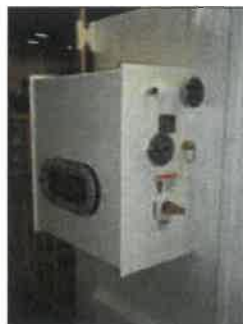
Figure 7. External visible break with gauges.
